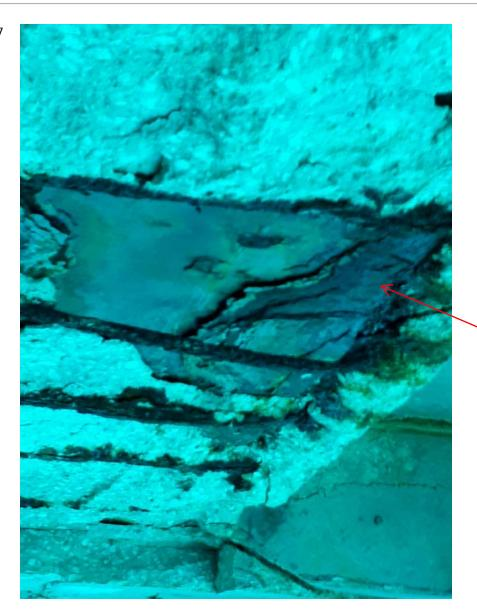
Rust pack on bottom flange of HP14x73 steel beam
