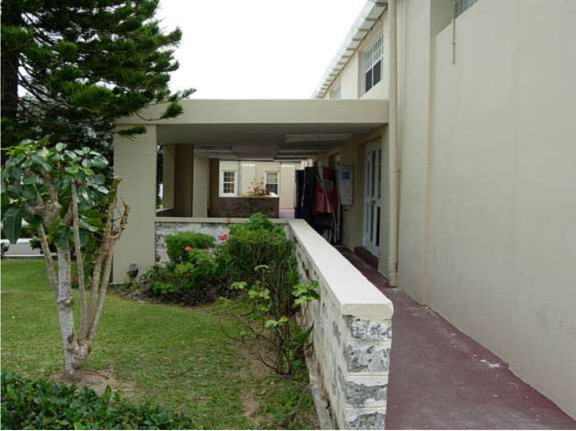
Porch Roof (East Elevation)
