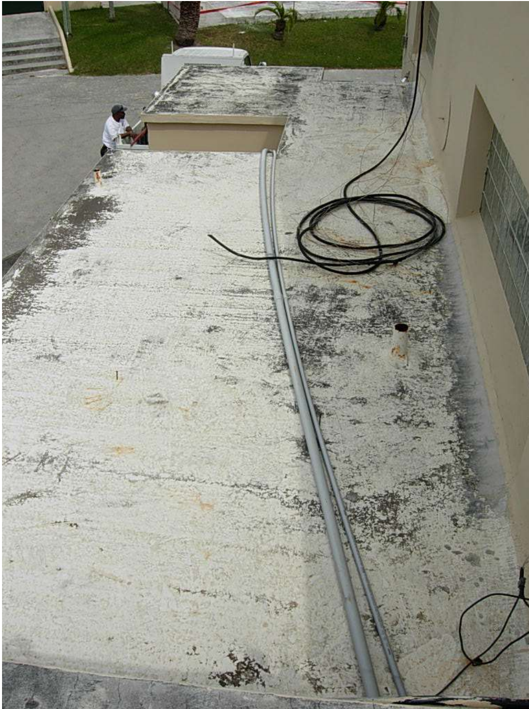
Storage Roofs (North Elevation)
