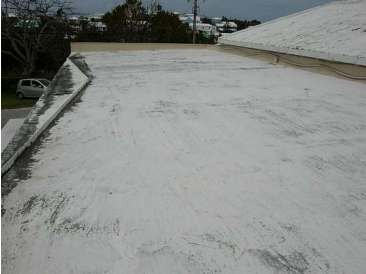
Medic, Kitchen and Dining Hall Roofs (West Elevation)
