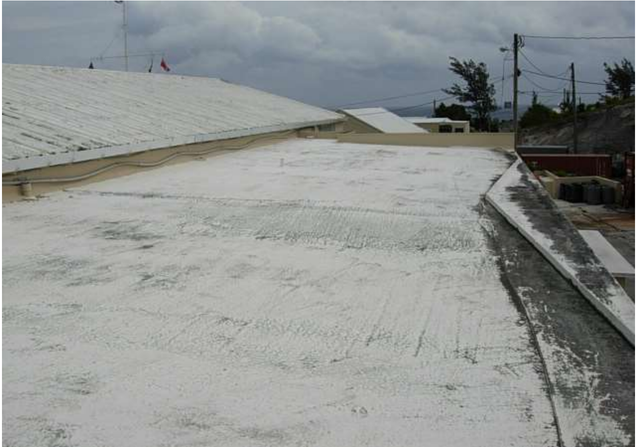
Medic, Kitchen and Dining Hall Roofs (West Elevation)
