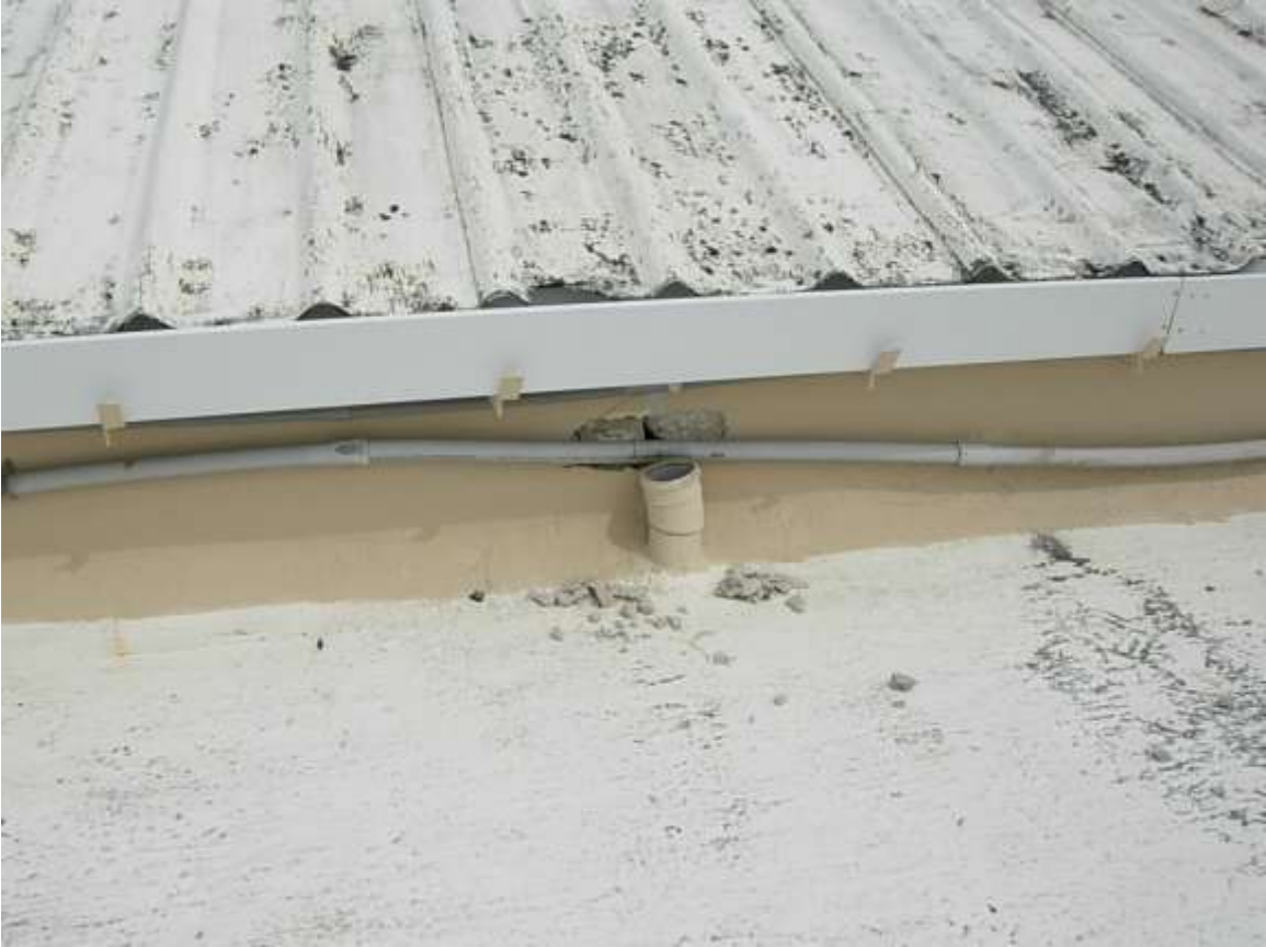
Up-stand and Gutter to Dining Hall Roof (West Elevation)
