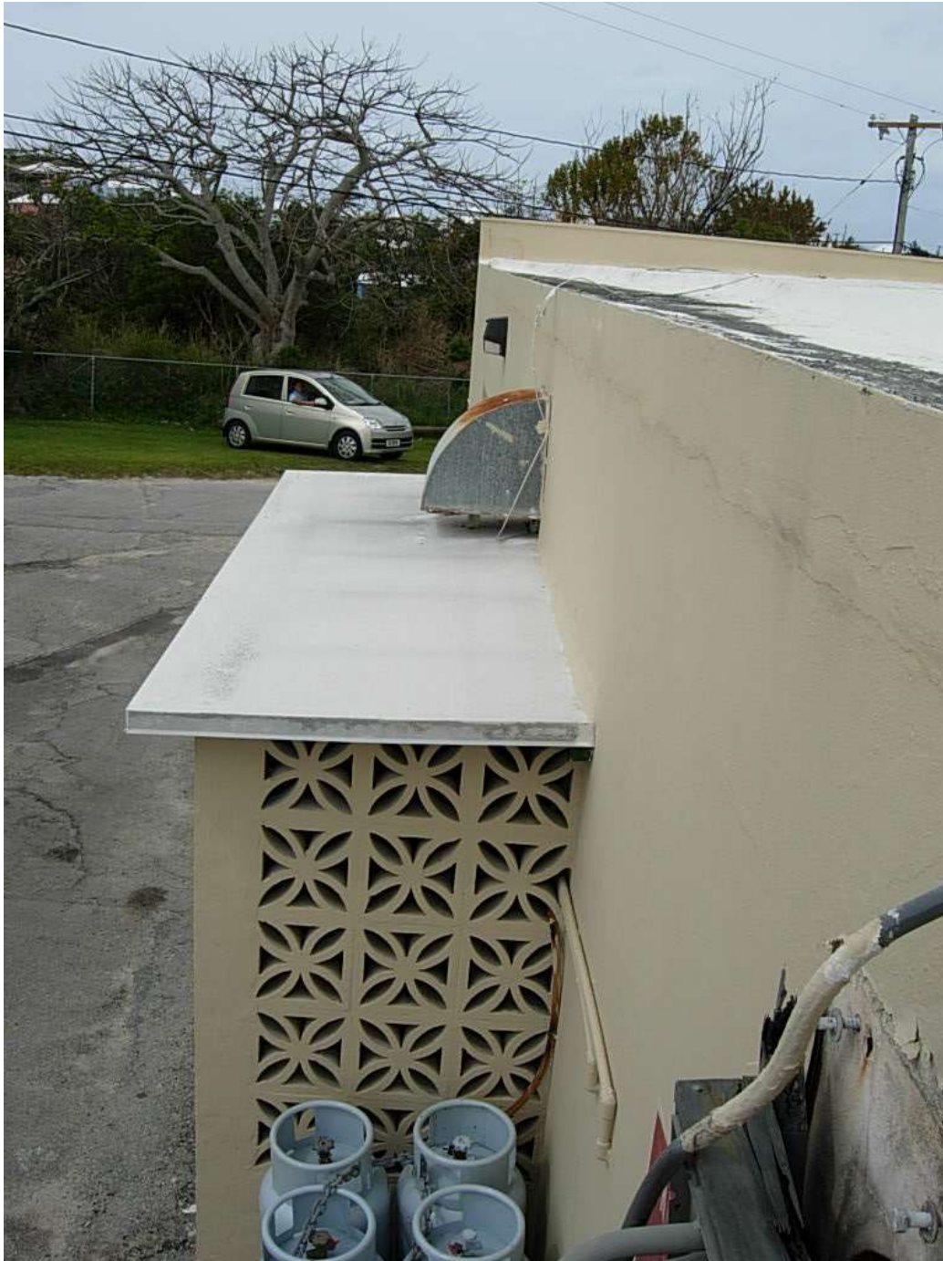
Porch Roof (West Elevation)
