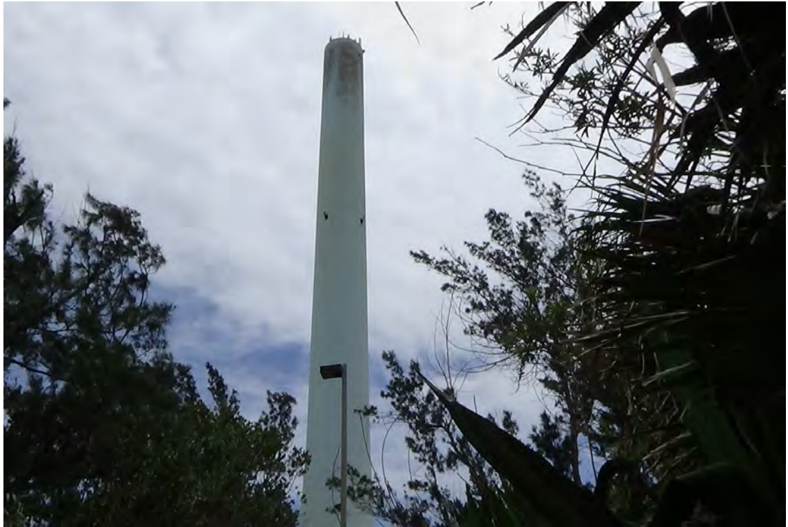
Overview of Tynes Bay 246' chimney. Inspections were performed inside both liners, ultrasonic thickness measurements were taken throughout the height of both liners. Exterior inspections were conducted on the north & south sides from a boatswain's chair. One annular inspection was performed from the access ladder.
