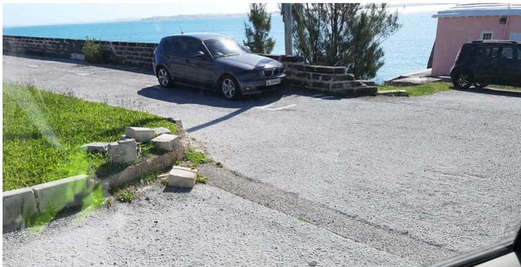
Figure 7. Additional broken kerb near Watford Bridge Ferry Terminal
