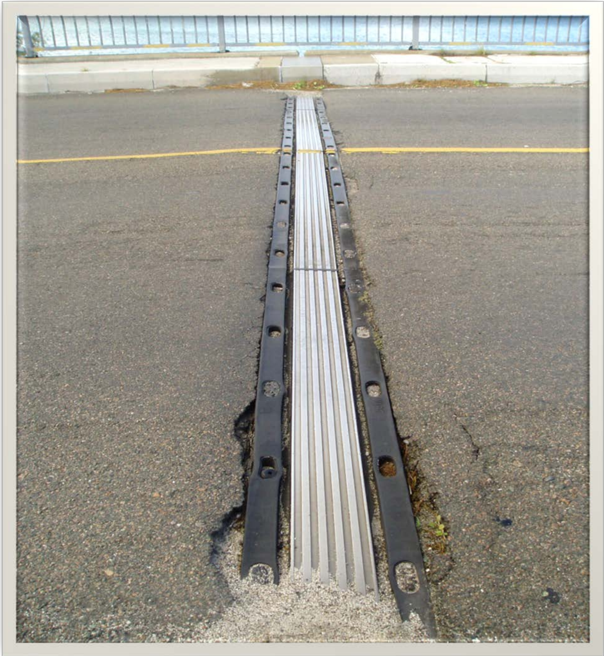
Figure 5: South Expansion Joint
