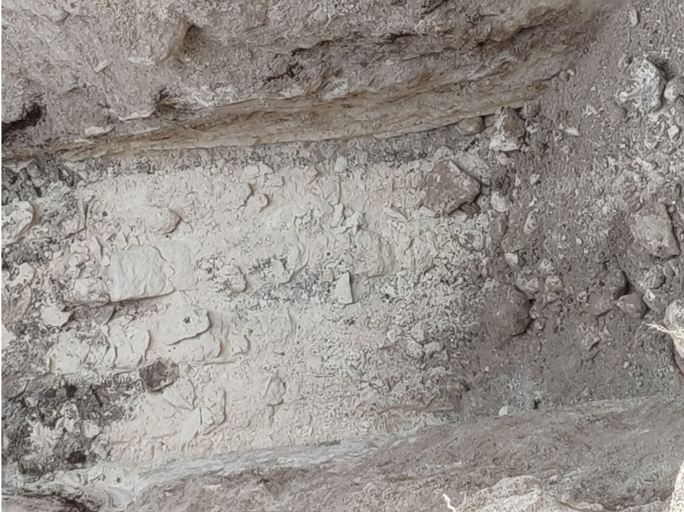
Trial Hole #2 – Excavation to prove rock
