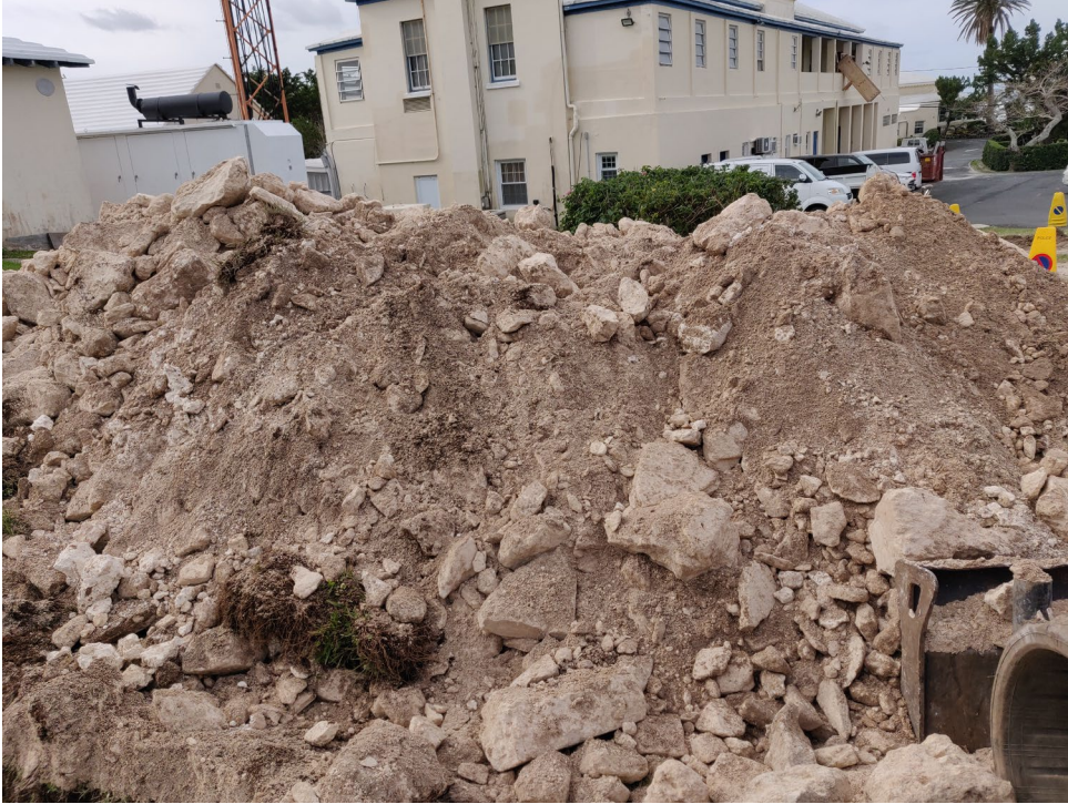
Trial Hole #2 – Arisings
