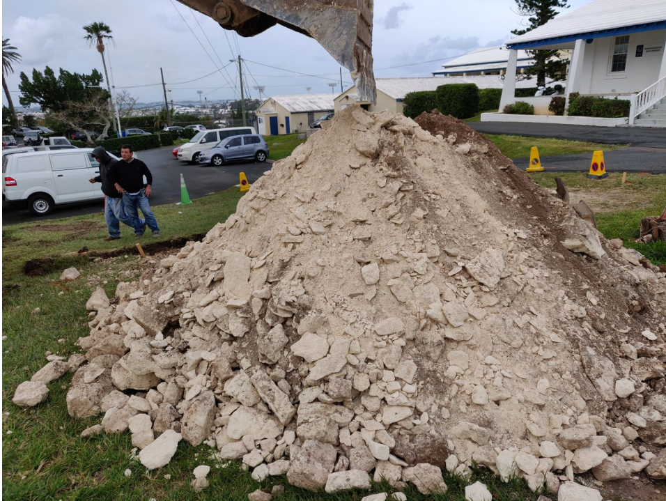
Trial Hole #1 - Arisings
