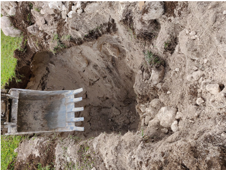
Trial Hole #2 – General fill material
