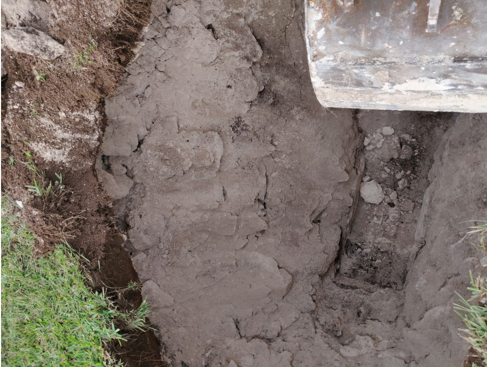
Trial Hole #2 – Rock level
