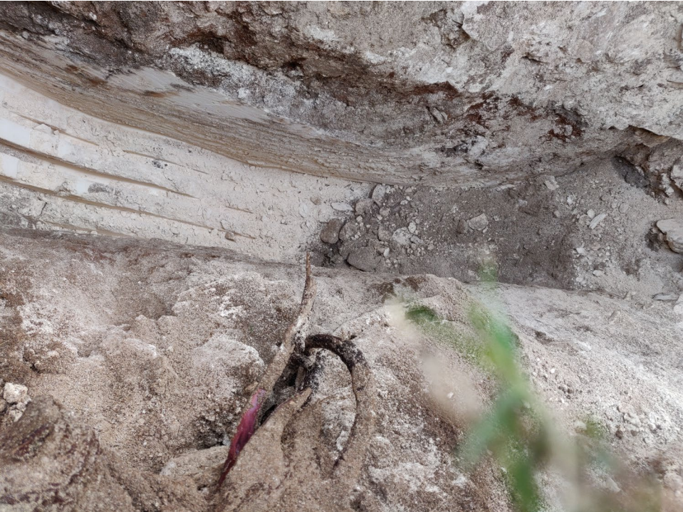
Trial Hole #1 – Excavation to prove rock
