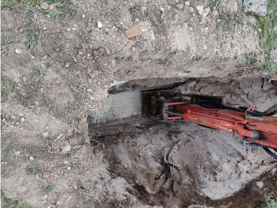
Trial Hole #1 – Rock Level
