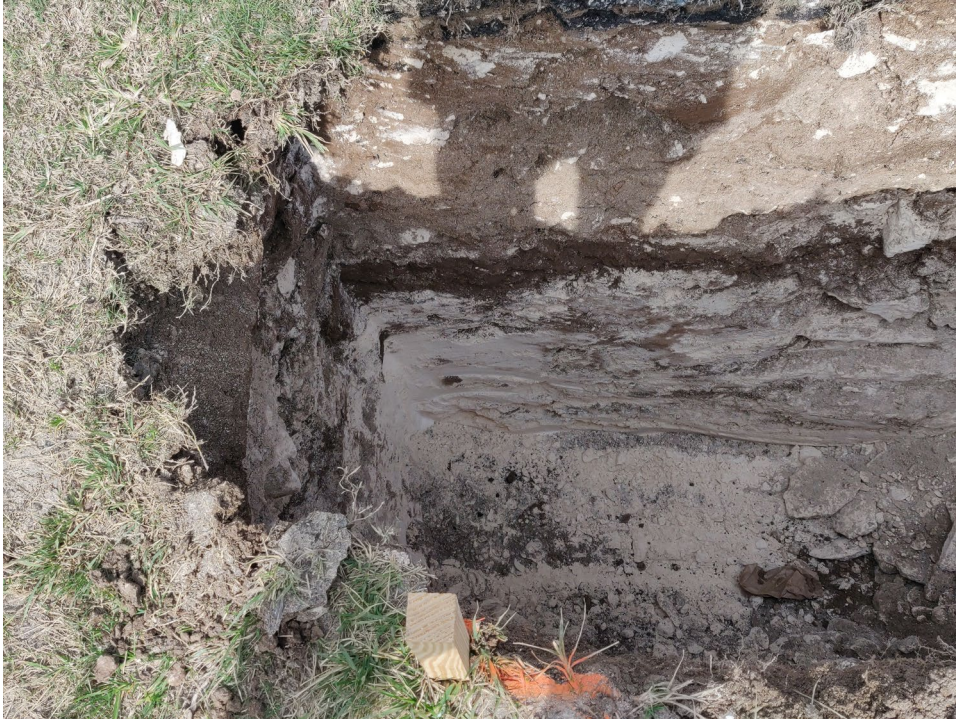
Trial Hole #3 – Excavation to prove rock
