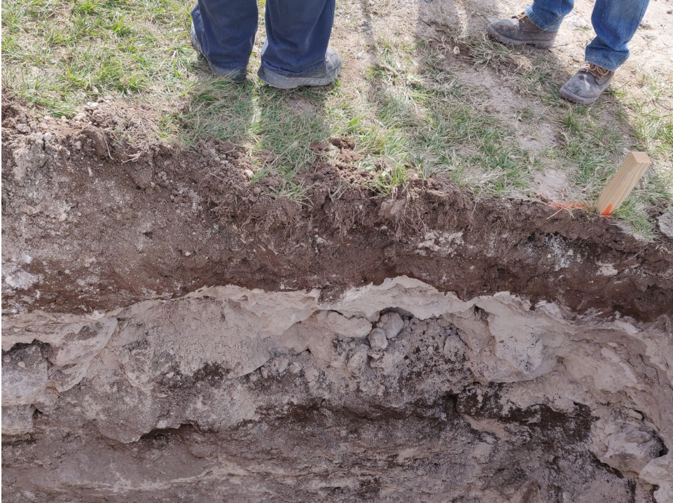
Trial Hole #3 – Topsoil and general fill
