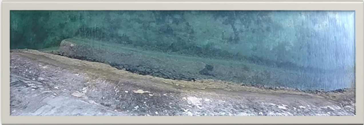
Figure 1: South East edge of landing located at Clarence Cove. View from top of landing.
