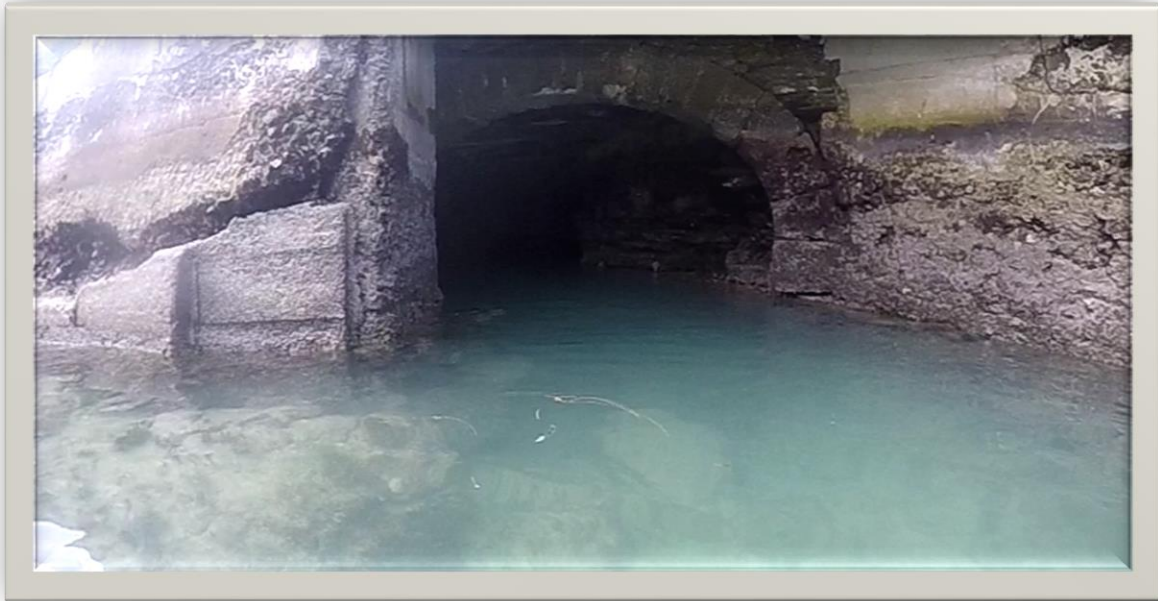
Figure 11: Arched pass though from South Face.
