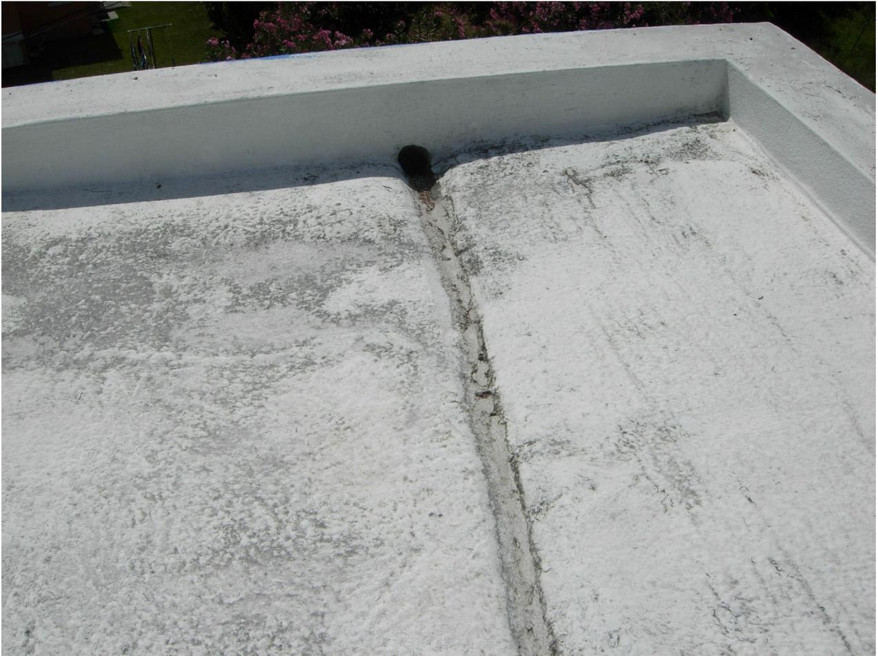
**Typical Rainwater Drainage Channel and Outlet (1 of 4)**
