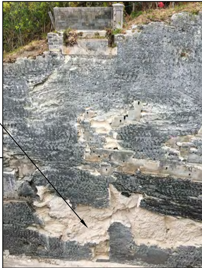
OVERVIEW PHOTO OF SHOTCRETE AREA
