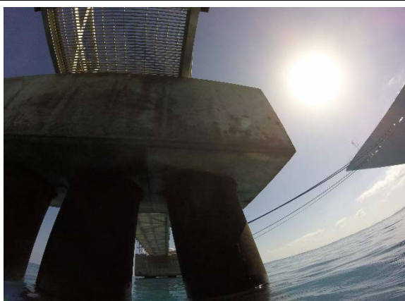
Fig. 3o General view of walkway dolphin
