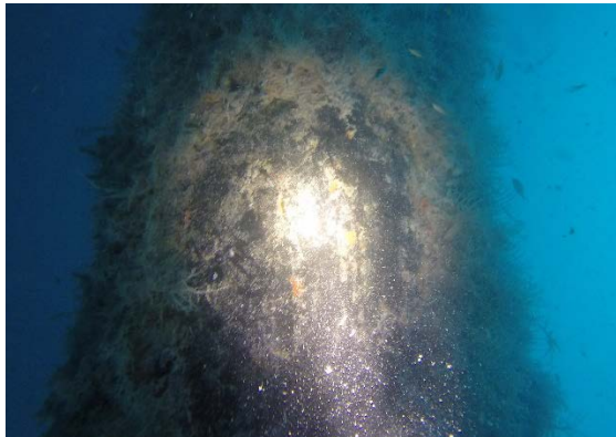
Fig. 1l 1 st Level 2 inspection, Pile 45, protective coating intact
