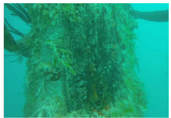
Fig. 3r - 2 nd Level 2 inspection, walkway dolphin
