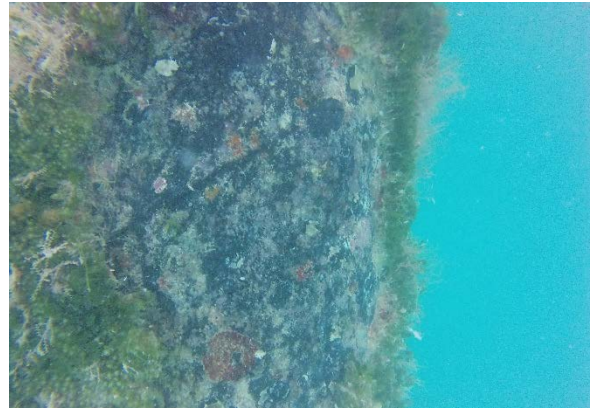
Fig. 2b 1 st Level 2 inspection, Pile 165
