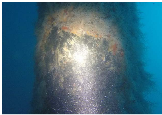
Fig. 1m 2 nd Level 2 inspection, Pile 45, protective coating intact
