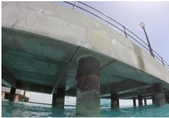
Fig. 2e – General view of Gangway splash zone
