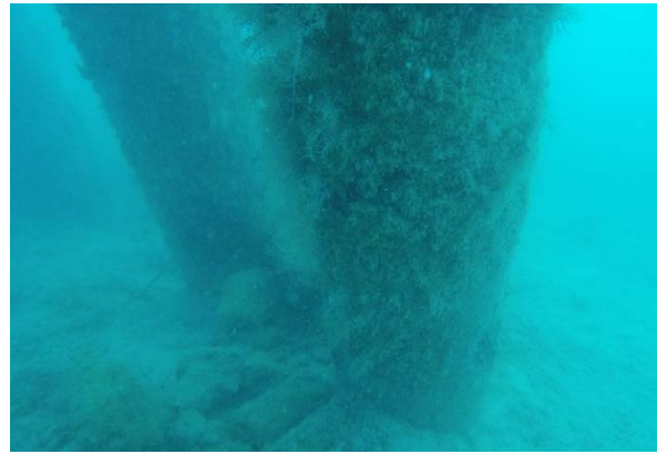
Fig. 3n Piles driven into sandy bottom, H-MD3
