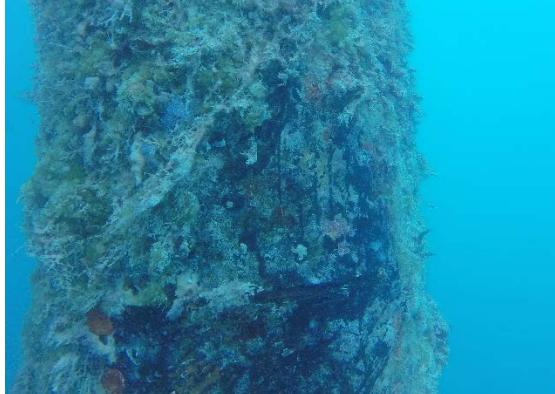
Fig. 1g - 3 rd Level 2 inspection, Pile 1
