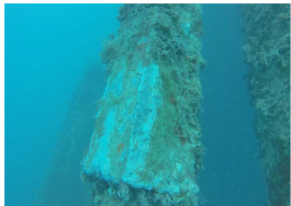
Fig. 3d - Level 2 inspection on anode, H-MD6
