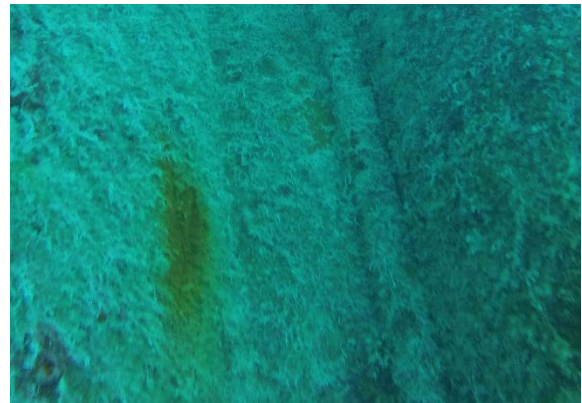
Fig. 2j - ALWC on metal sheet pile
