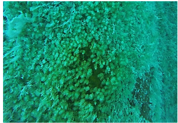
Fig. 2h - ALWC on metal sheet pile of North Arm
