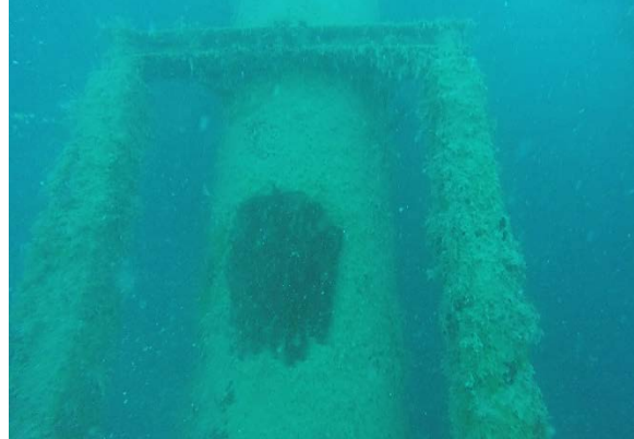
Fig. 3t – Anode and Level 2 inspection on H-BD3
