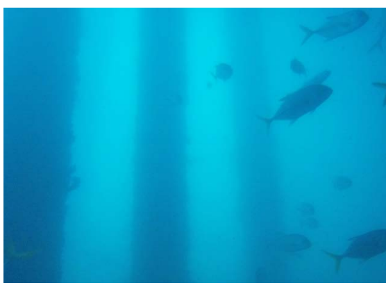
Fig. 1o General view of three of the piles from Cluster 2
