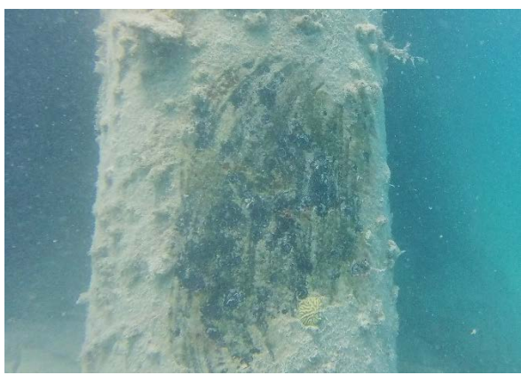
Fig. 3ff - Level 2 inspection, H-MD1, protective coating still intact.
