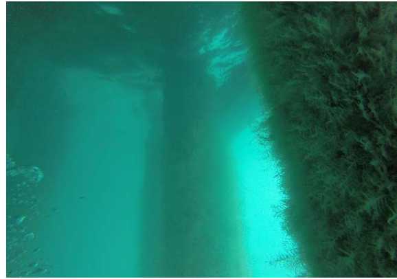
Fig. 1k Cluster 1 composed of 6 piles
