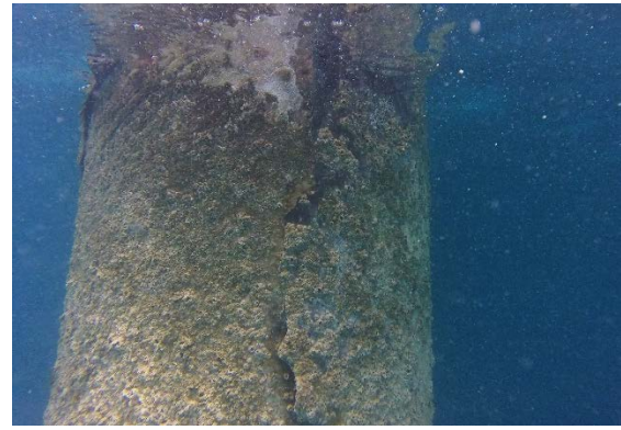
Fig. 1w – Just below surface, Pile 66
