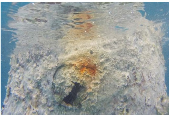
Fig. 1h - ALWC near high water mark
