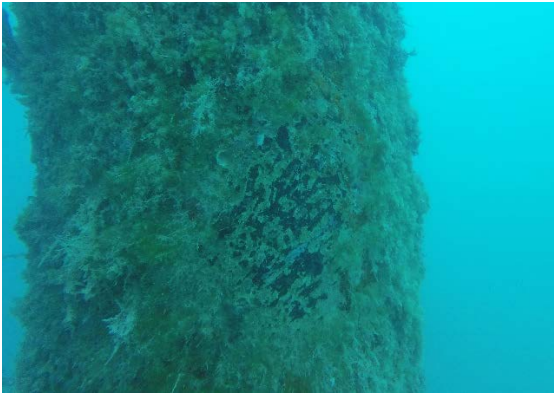
Fig. 1f - 2 nd Level 2 inspection, Pile 1
