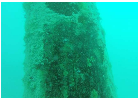
Fig. 3q - 1 st Level 2 inspection, walkway dolphin
