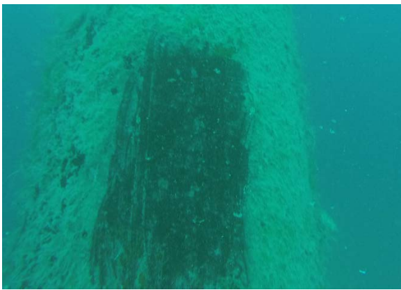
Fig. 3u - Level 2 inspection, H-BD3
