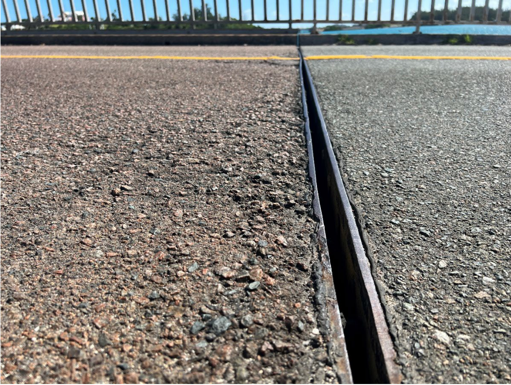
Photograph 1 – Existing end plates
