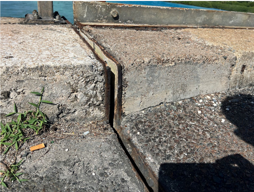
Photograph 2 – End plate at curb location
