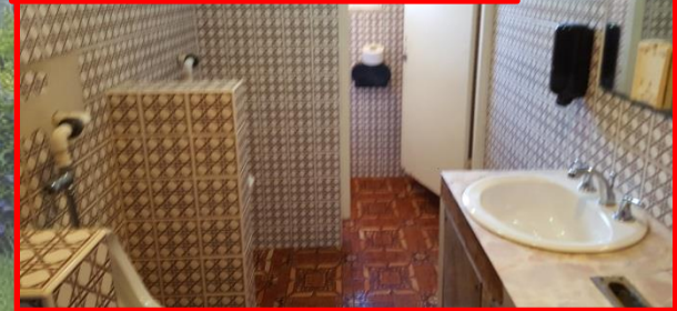
Visitor's Centre: Men's Bathroom
