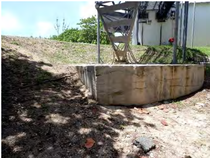
Tower foundation Photo File 19
