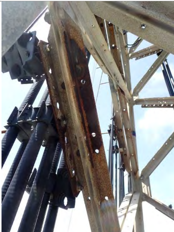
Tower surface condition Photo File 63
