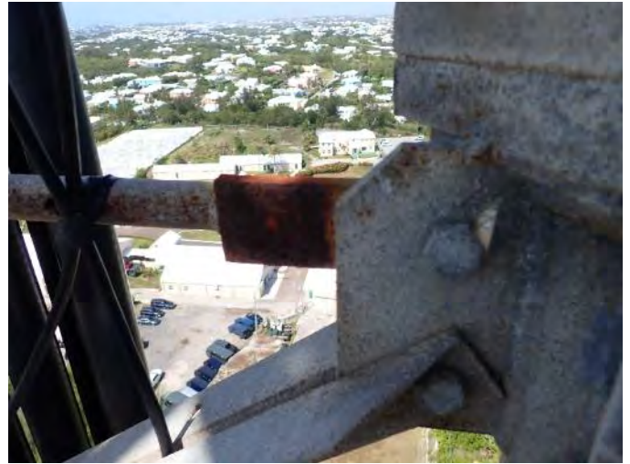
Tower surface condition Photo File 134
