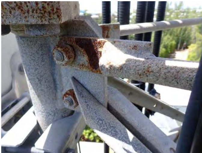
Tower surface condition Photo File 43
