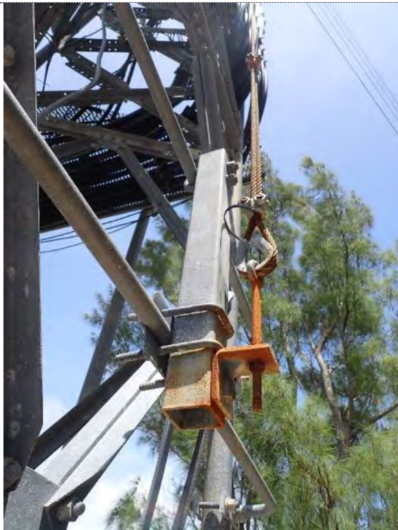
Safety cable bracket Photo File 23
