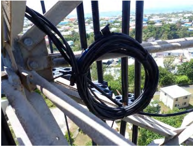
Abandoned feedlines Photo File 81
