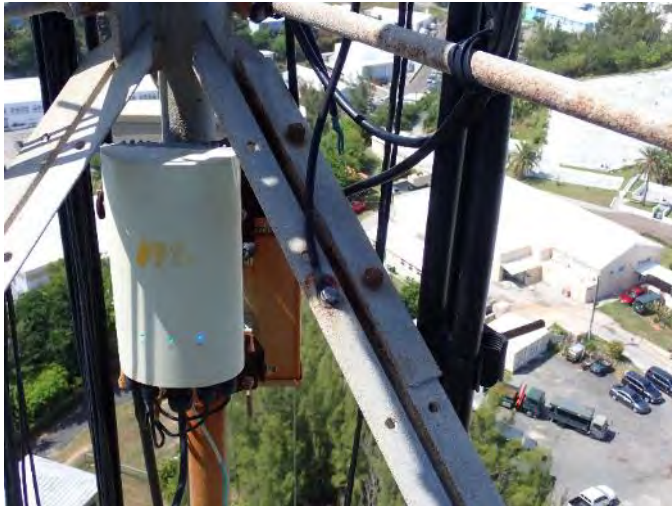
Tower surface condition Photo File 135
