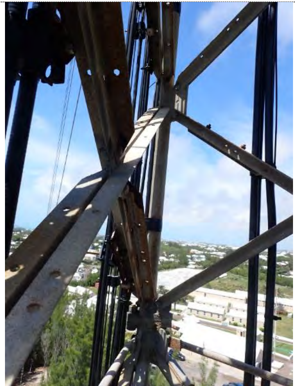
Tower surface condition Photo File 64
