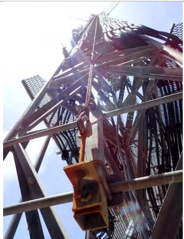
Safety cable bracket Photo File 24
