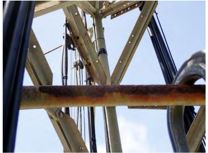
Tower surface condition Photo File 48
