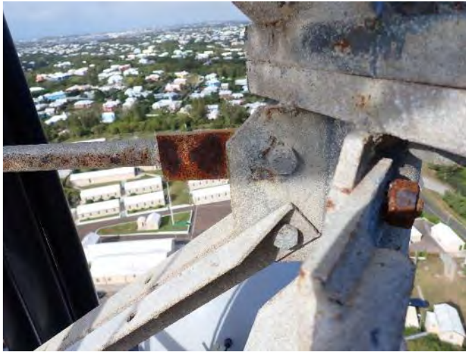
Tower surface condition Photo File 217
