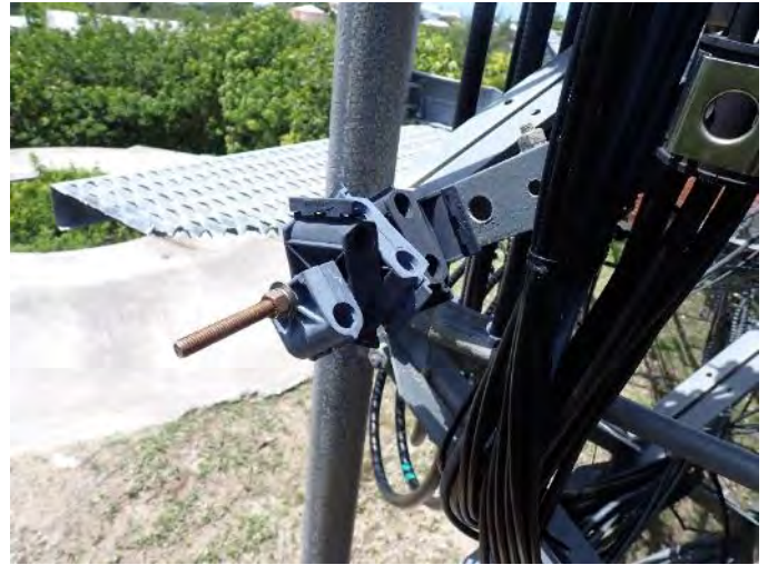
Abandoned feedline hangers Photo File 26
