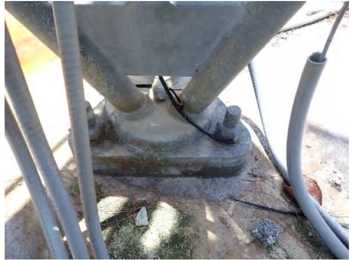
Tower base Photo File 22
