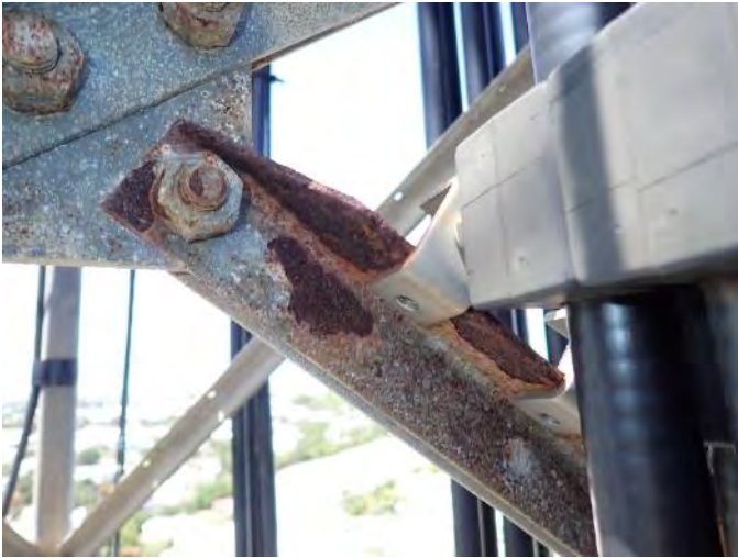
Tower surface condition Photo File 71
