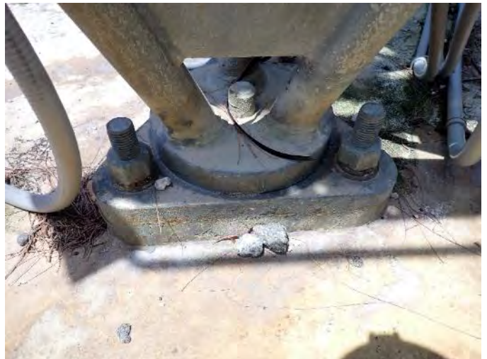
Tower base Photo File 20
