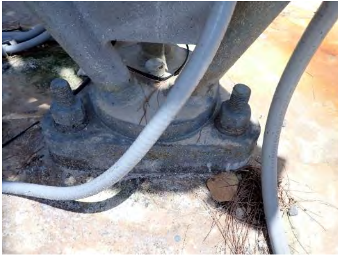
Tower base Photo File 21
