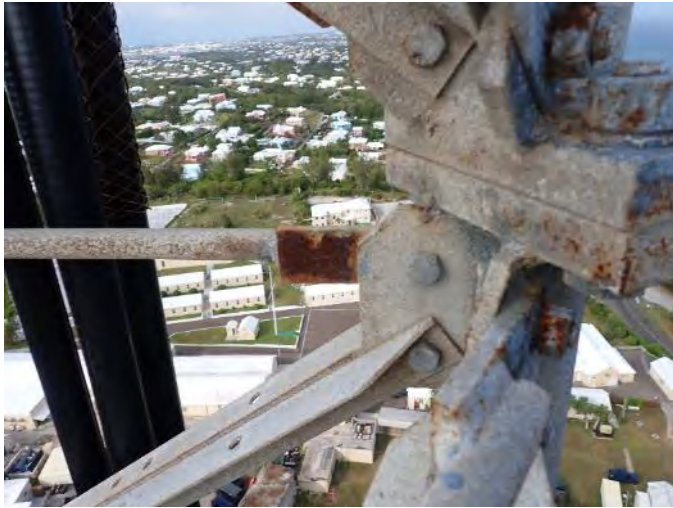
Tower surface condition Photo File 225
