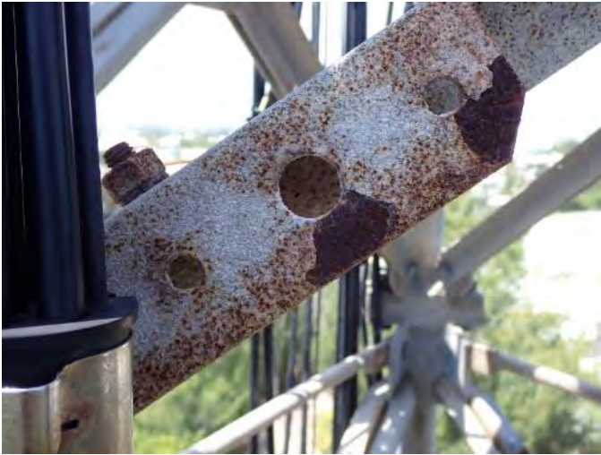
Tower surface condition Photo File 49
