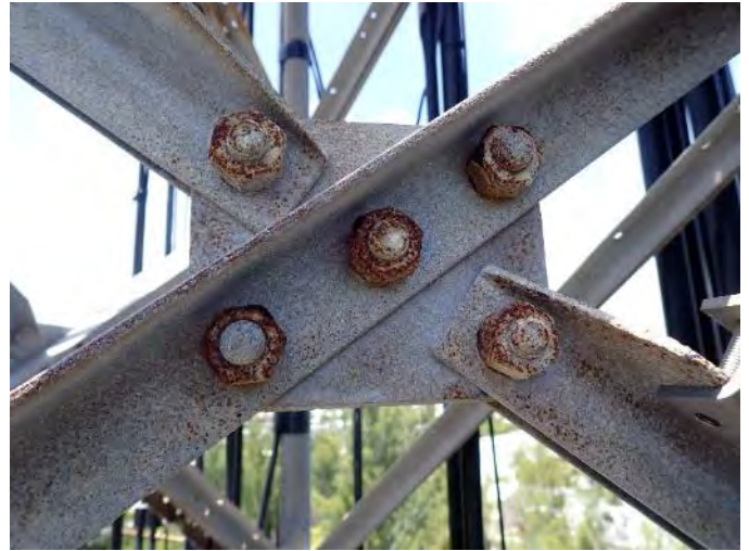
Tower surface condition Photo File 42
