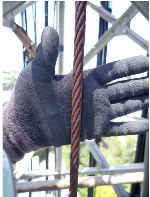
Safety cable condition Photo File 62
