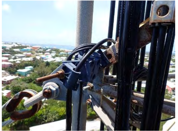
Abandoned feedlines Photo File 82
