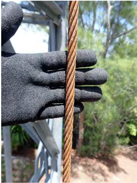
Safety cable condition Photo File 25
