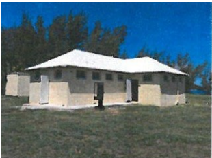
4 View from Southeast View from Southeast MTS
