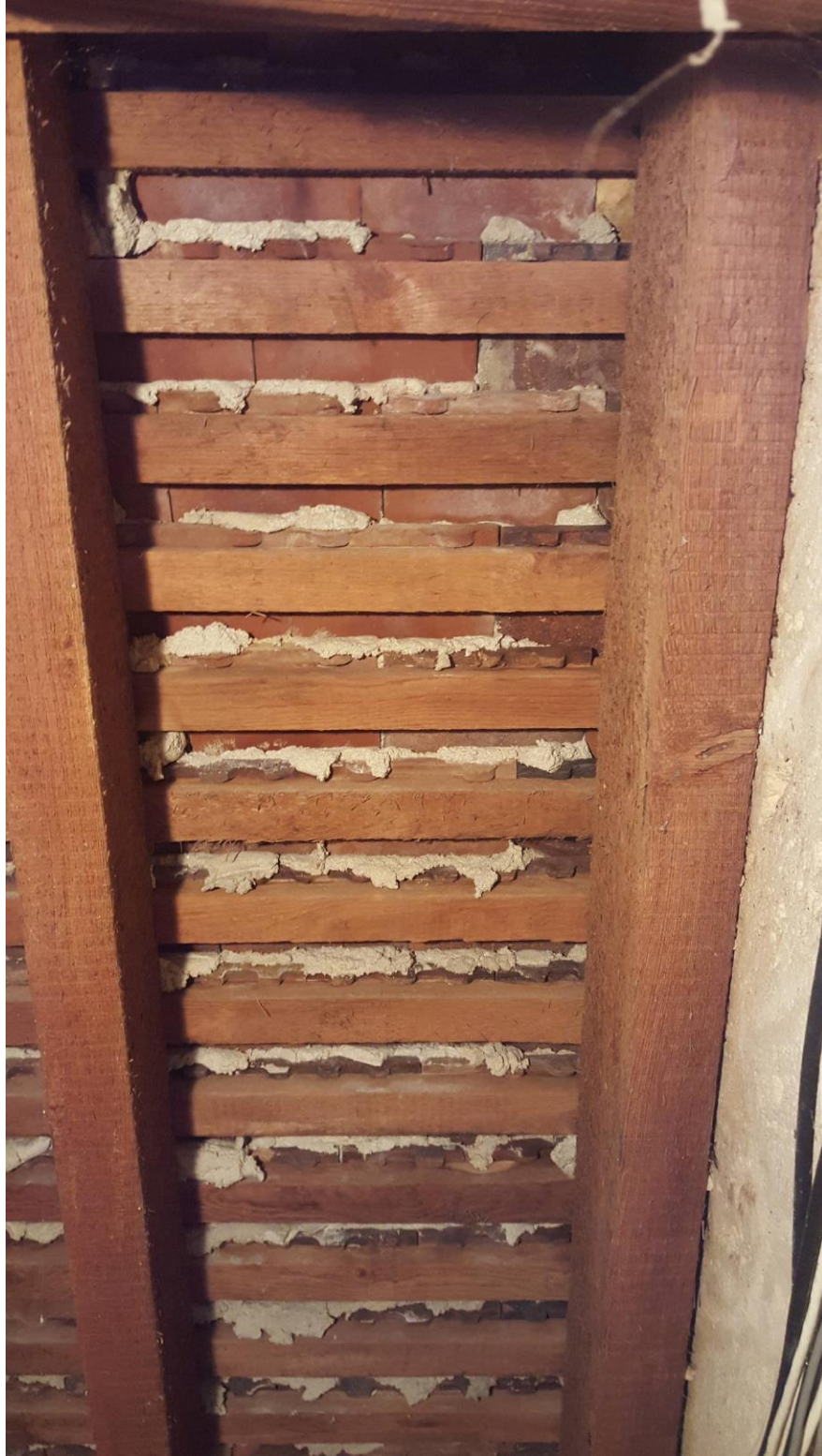
Underside of Existing Clay Tile Roof Coverings
